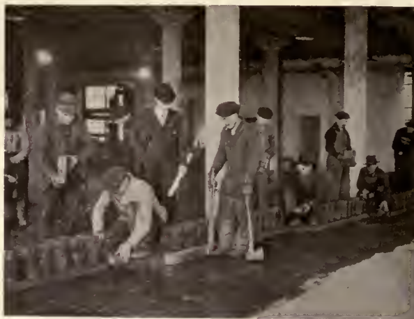
LAYING A WOOD BLOCK FLOOR
